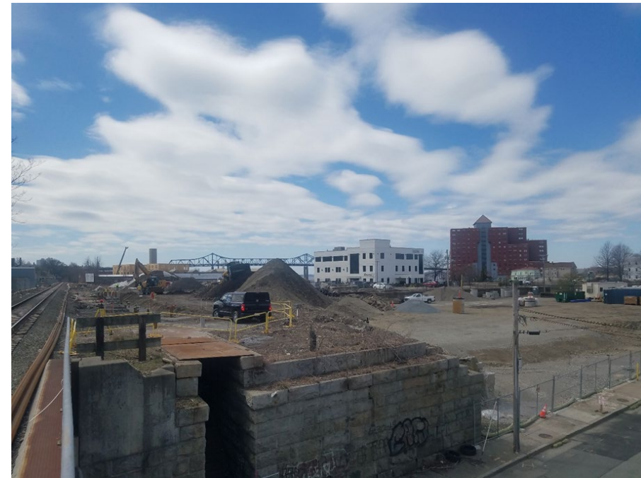
Fall River Depot – general view looking south
