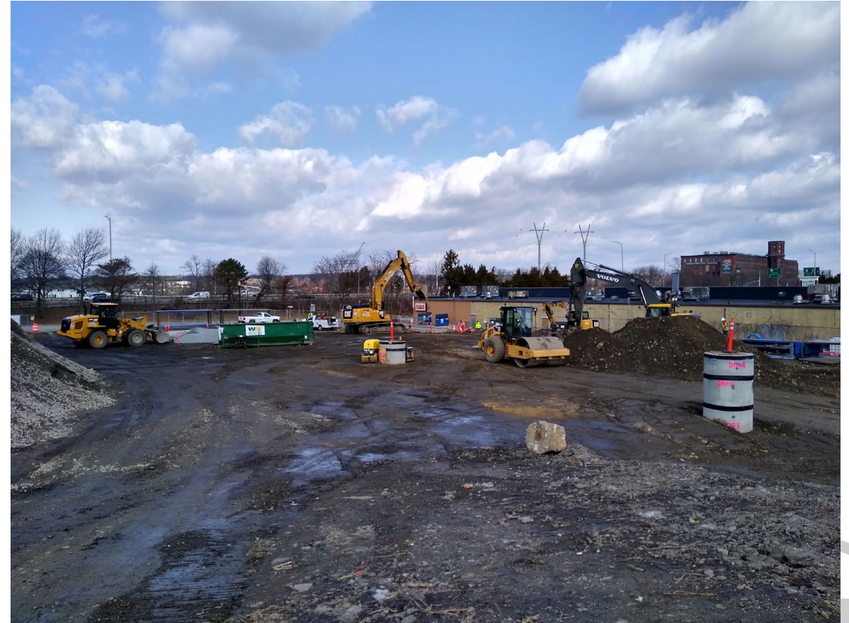
Heavy equipment work at Fall River Depot
