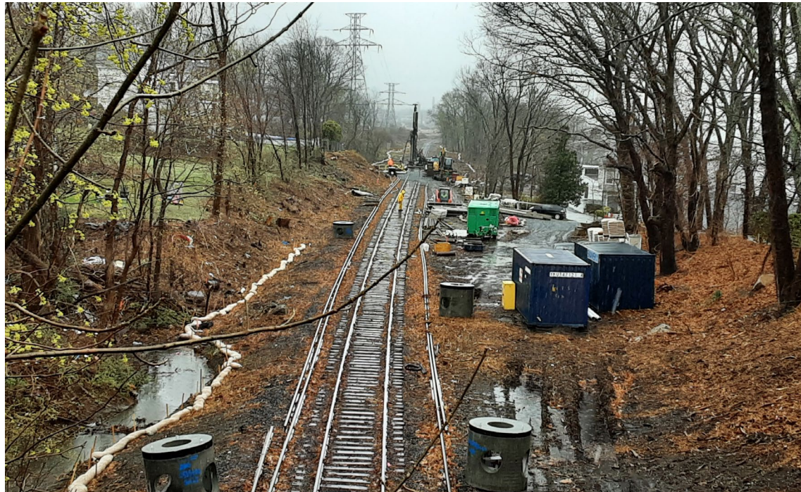
Clark Street Bridge – looking south to Collins Street
