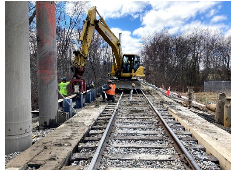
Hub Foundation Soldier piles at Wall S
