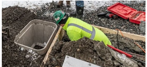
Upgrade a Traction Power Substation
