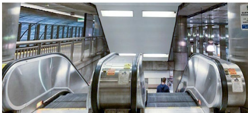
Oak Grove: modernize three escalators to improve station accessibility, replace 1,180 track ft, and enhance station
