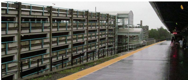
Repair parking lot pavement at multiple parking facilities (systemwide)
