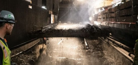
Complete repair of 32,000 feet of track (6 miles, including concrete track foundations)
