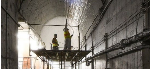
Tunnel leak mitigation between Alewife - Harvard Stations
