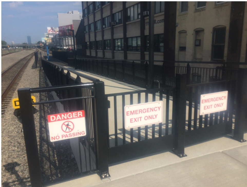
Photo: Example ramp to area of rescue assistance, “holding pen.”
